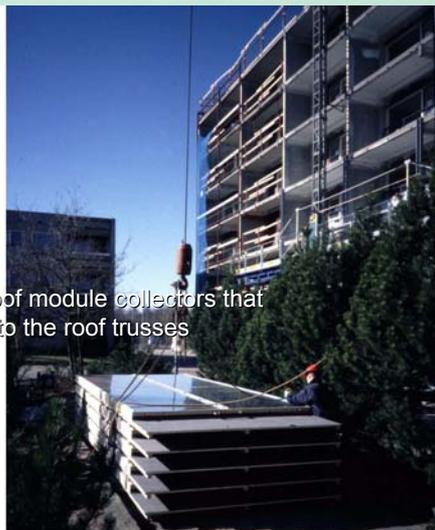
Roof module collectors that fit to the roof trusses
